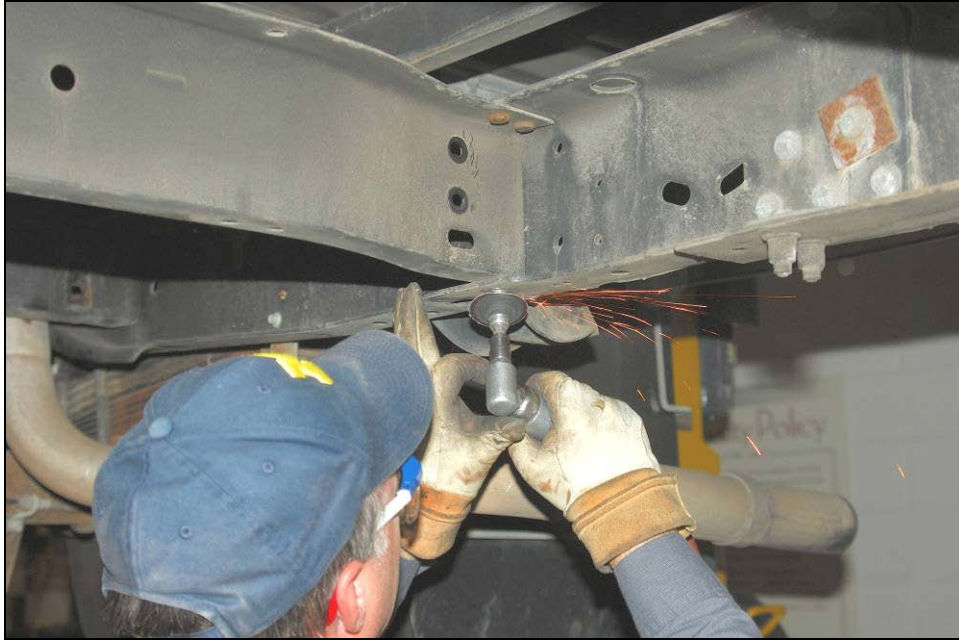
Trimming Lower Rear Crossmember Rivet
