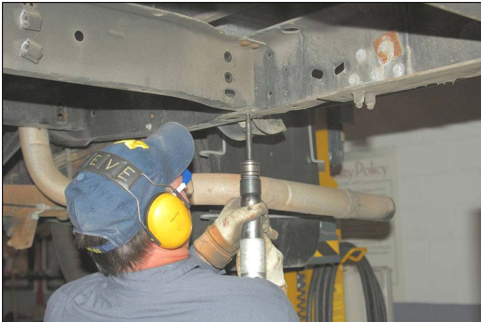
Punching Out Rear Crossmember Rivet
