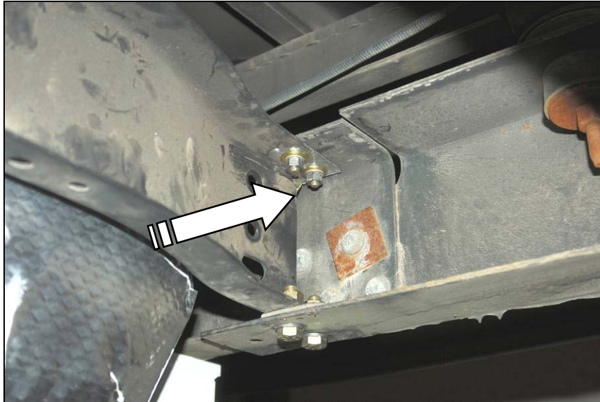
Area of Rear Crossmember Modification
