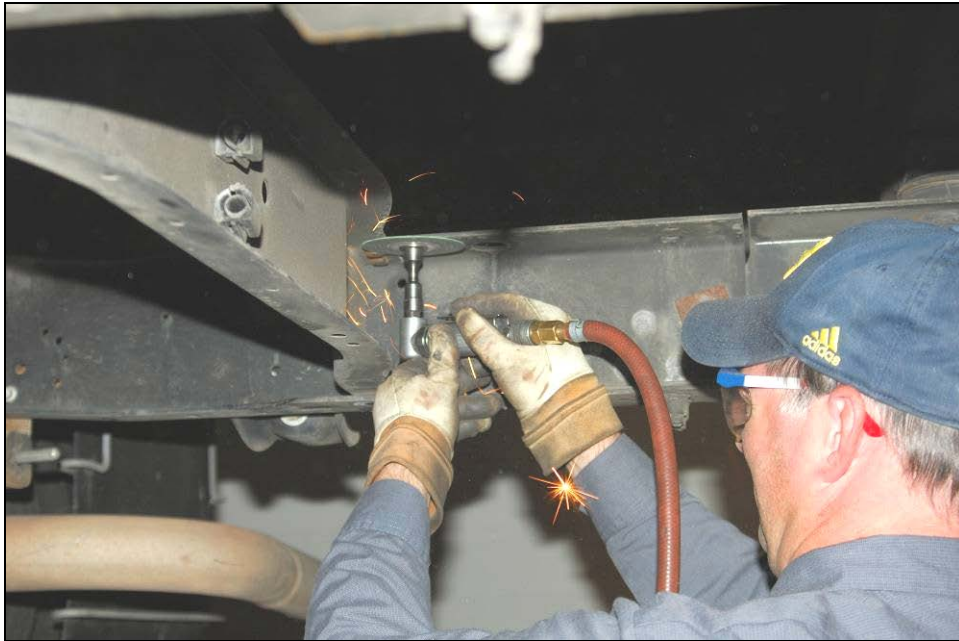
Grinding Upper Rear Crossmember Rivet
