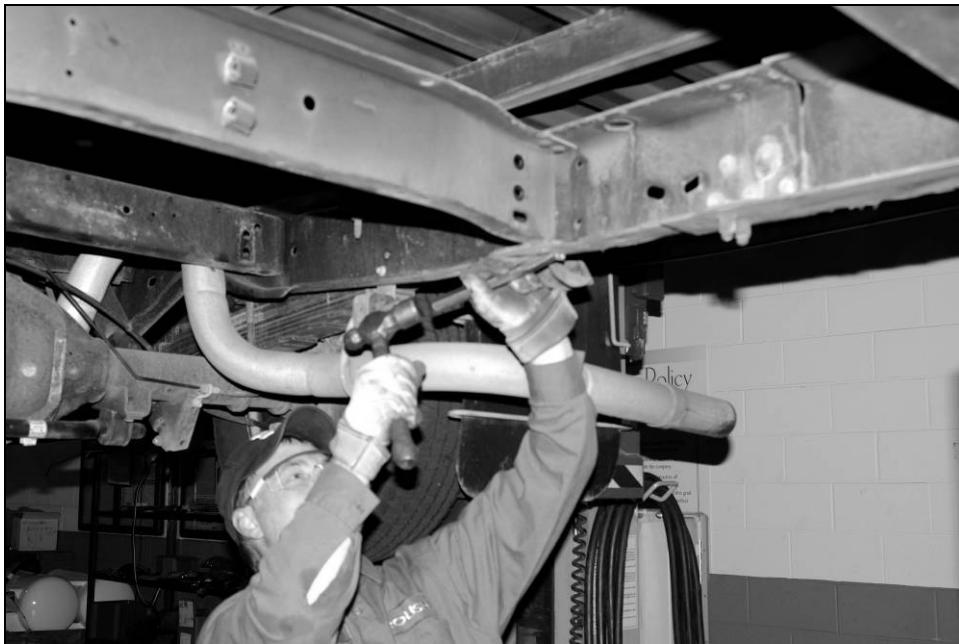
Chiseling Lower Rear Crossmember Rivet
