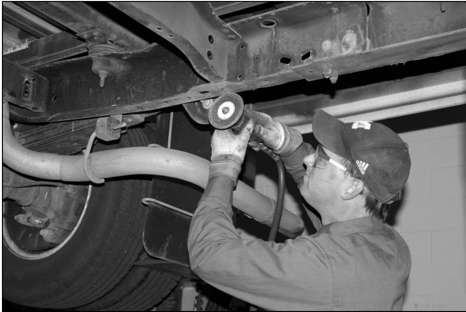
Cutting Lower Rear Crossmember Rivet
