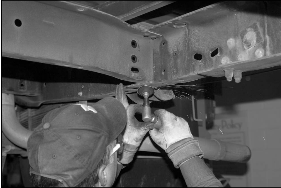
Trimming Lower Rear Crossmember Rivet
