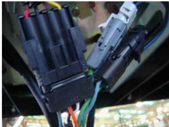
Figure 41 – Fuel Tank Connectors
