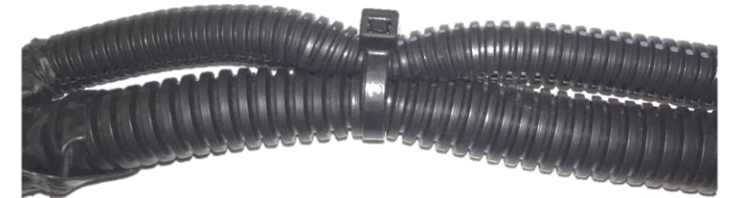
Zip-tie fastened too TIGHT
