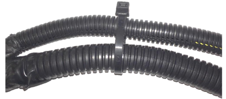
Zip-tie fastened too LOOSE
