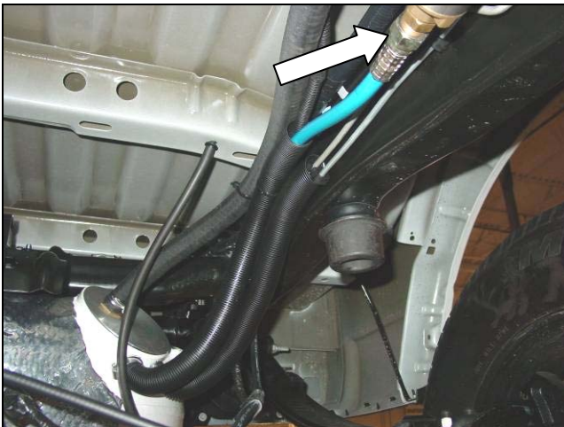
Figure 67 — Fuel Fill Line at Filter Outlet
