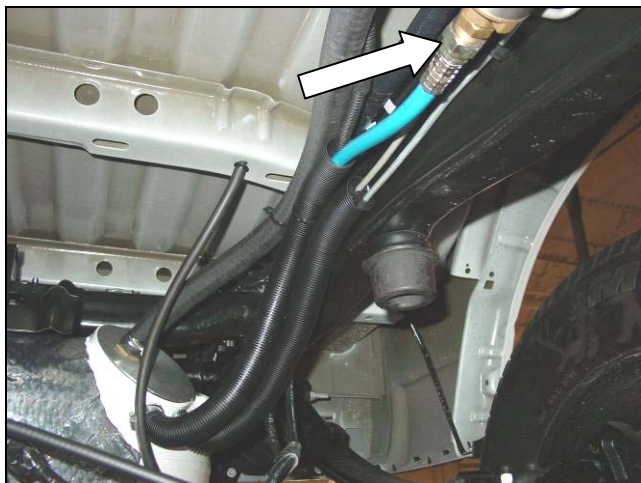
Figure 53 — Fuel Fill Line at Filter Outlet
