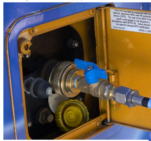
Figure 6. OPEN Ball Valve Connection to Donor Tank
