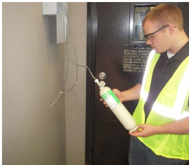
Figure 30. Gas detector calibration tubing. Photo from Gladstein, Neandross & Associates, NREL 44684
