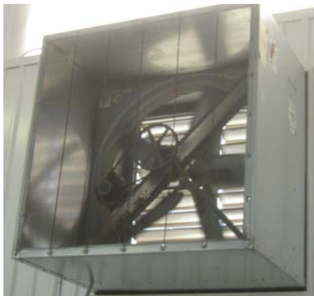
Figure 16. Powered sidewall fan that provides make-up air flow. Photo from Gladstein, Neandross & Associates, NREL 44707
